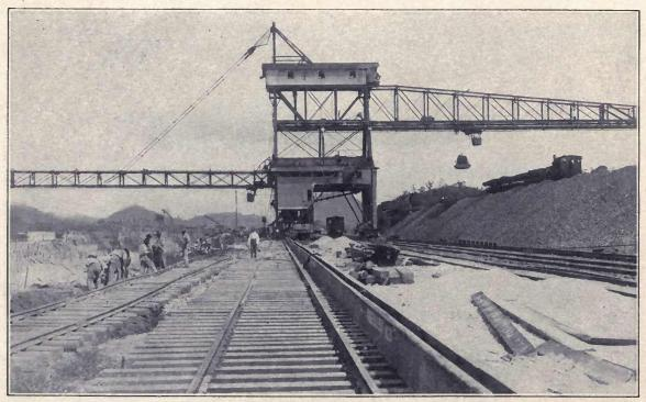
A View of one of the Berm Cranes as they appear at Miraflores. They are used for Mixing and Conveying Concrete
